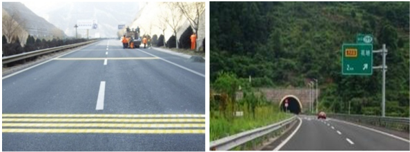
图 7 减速带实物图 Fig.7 General view of road continuous speed bumps
